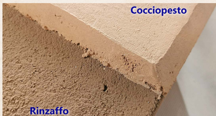
Rinzaffo MGN and Cocciopesto MGN plaster for basements
