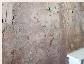
Dark patches: insufficient thickness
